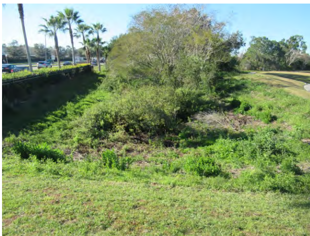
Sediment accumulation (Pond 21 shown)
