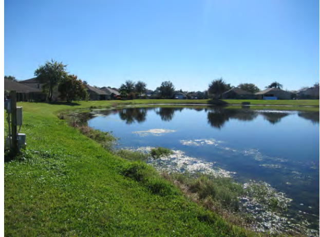
Debris accumulation and weed growth (Pond 4 shown)
