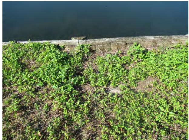
Minor soil erosion behind bulkhead (Pond 1 shown)
