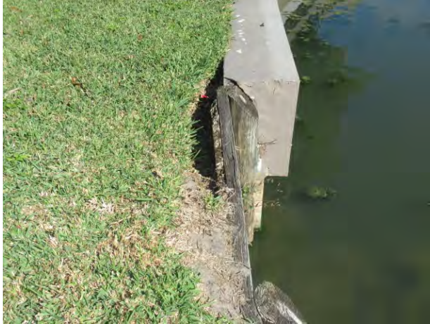
Soil erosion behind bulkhead (Pond 23 shown)
