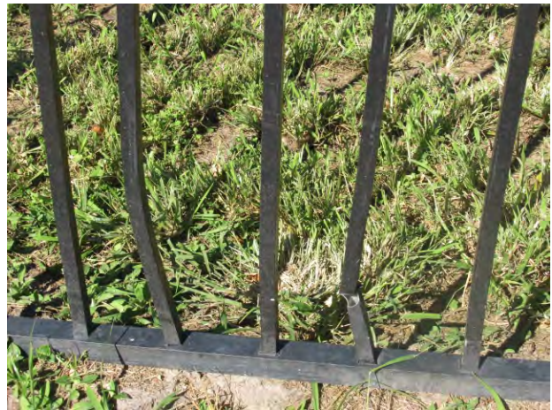
Damaged fence pickets
