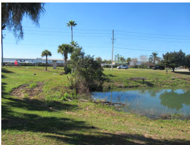
Overgrown vegetation and soil erosion (Pond 12 shown)
