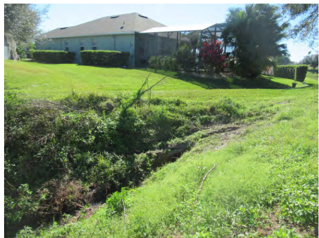
Sediment accumulation (Pond 6 shown)
