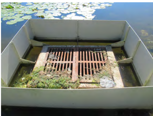
Structure partial covered by debris (Pond 2 shown)
