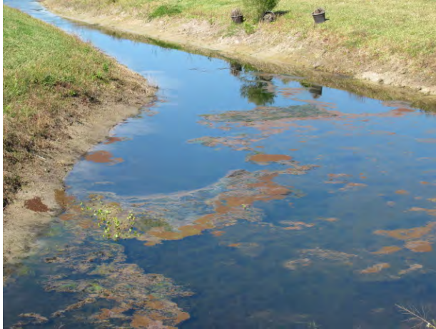
Debris accumulation (Pond 6 shown)
