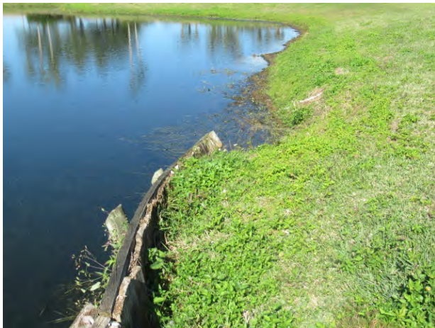
Minor movement and timber deterioration (Pond 1 shown)
