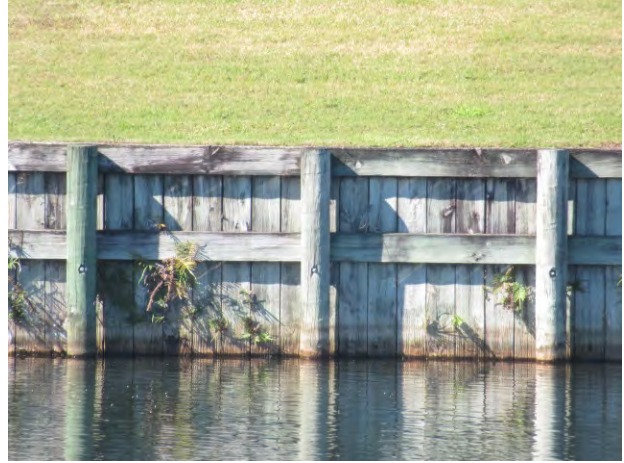
Timber bulkhead detail (Pond 1 shown)
