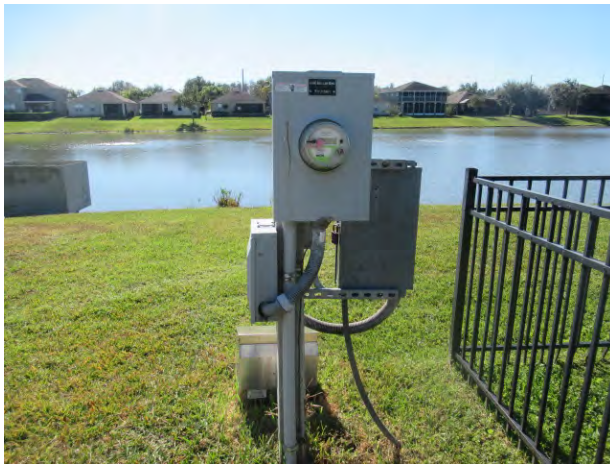
Typical aerator electrical panel
