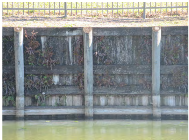
Bulkhead detail, note weathered wood and overgrown vegetation (Pond 23 shown)
