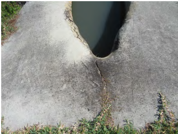
Minor concrete deterioration at structure connecting Ponds 6 and 7
