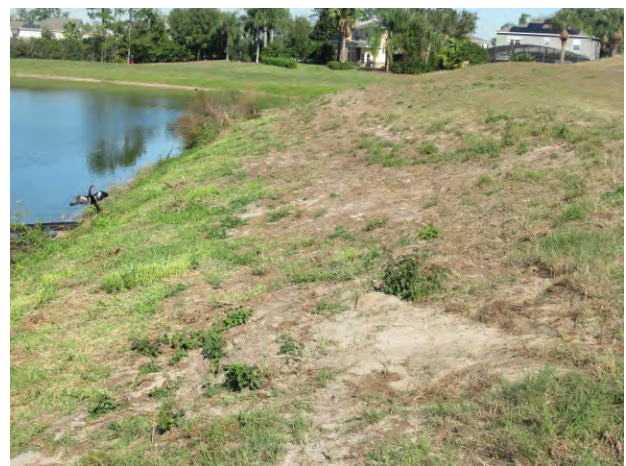
Soil erosion (Pond 14 shown)
