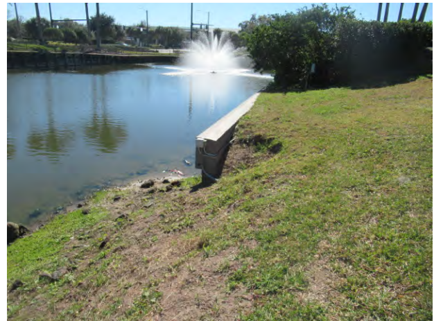
Soil erosion (Pond 23 shown)
