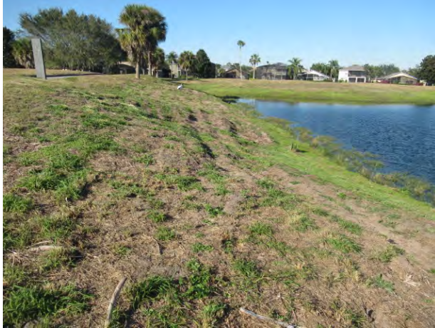
Soil erosion (Pond 17 shown)
